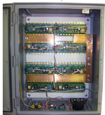
Interior view of enclosure
